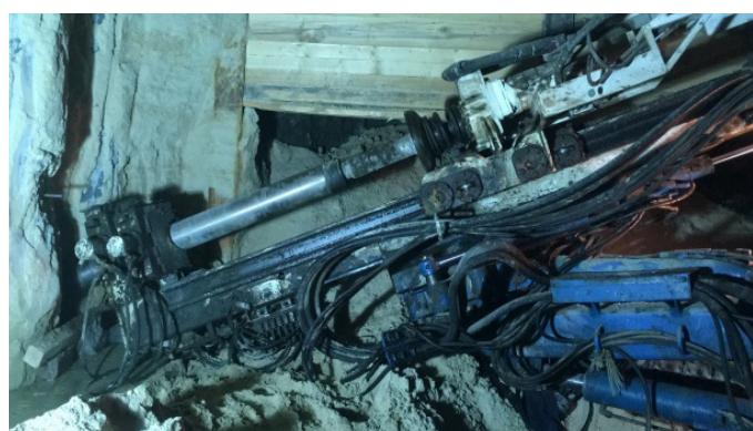
*ancillary and supporting equipments. For the execution of the contiguous piles of shoring by CAP (Cased Augered Pile), TFK had mobilized the drilling rig **Soilmec SR-100**) with 16 m long attached casing.*
